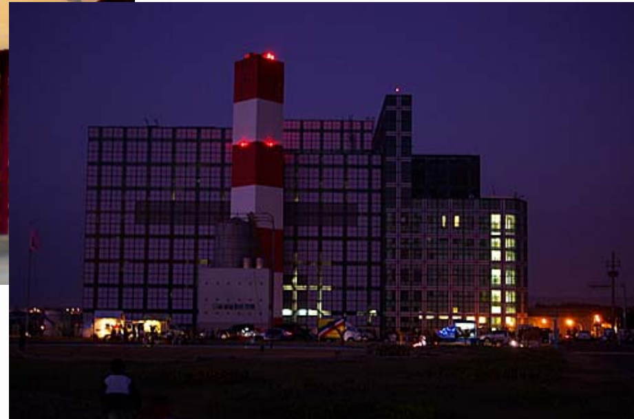
Location in NanLiao, Wasteyard
